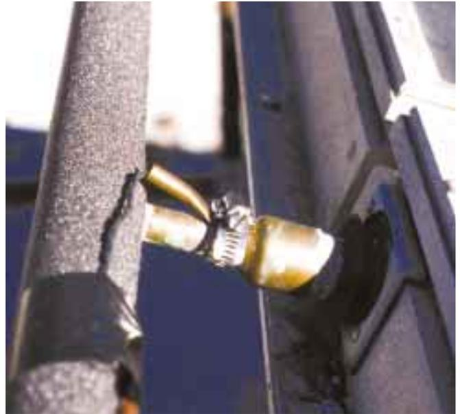
**A sensor measures temperature of water leaving the collectors. Another measures tank temperature.**
