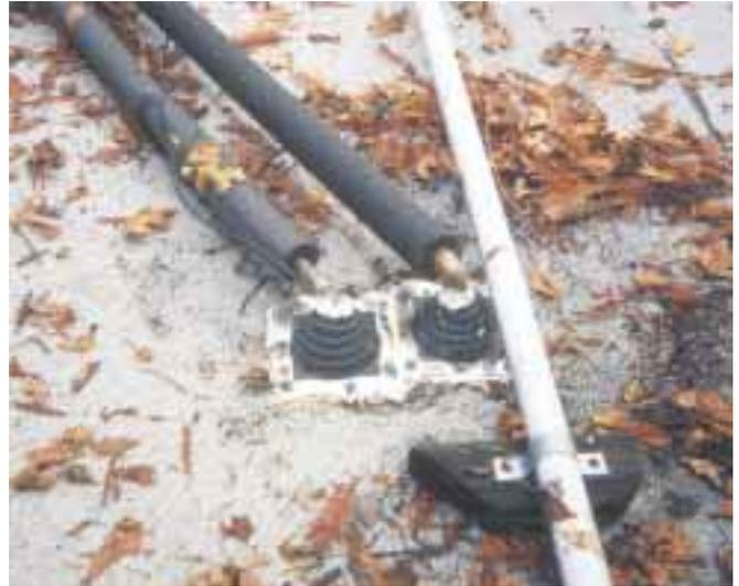
**Two sheet metal roof jacks with neoprene boots make roof penetrations weatherproof.**
